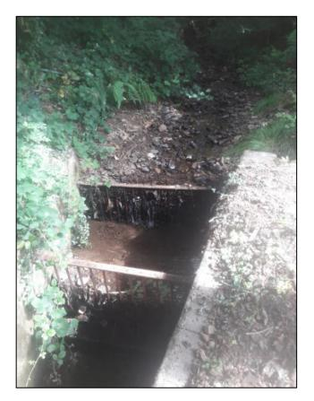
**Figure 23**: Photo of significant debris accumulation behind the upstream debris screens above 'Culvert Inlet 3' in the Nant Tyle-du watercourse (captured by a Council appointed contractor on 03/08/2020 during CCTV survey operations)
