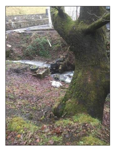
Figure 20: Image of tyre damn acting as an obstruction to the watercourse upstream of 'Culvert Inlet 2' (captured by RCT's Flood Risk Management team on 17th February 2020)
