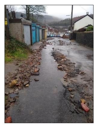
Figure 27: Road damage and debris deposited along Column Street by the surcharging ordinary watercourse flows during the storm event (image provided by resident)
