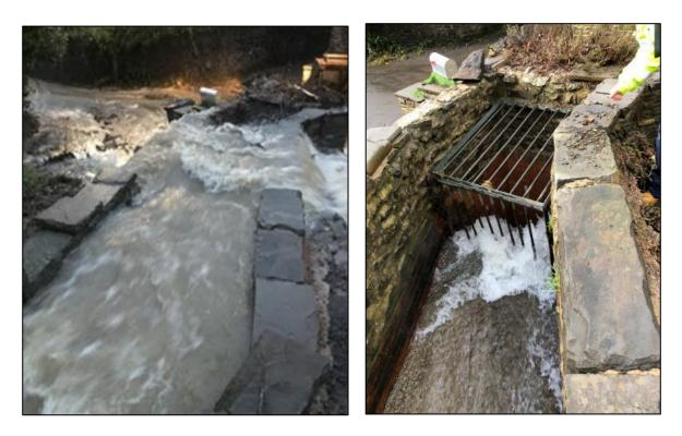
**Figure 5**: Evidence of 'Culvert Inlet 1' surcharging during the storm event and conveying southwards towards Column and Dumfries Streets (left) (image provided by resident), and 'Culvert Inlet 1' post storm event (right) (captured by RCT's Flood Risk Management team on 20<sup>th</sup> February 2020)
